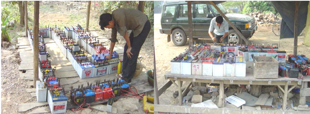
Picture 8: The battery acid is easily spilled onto the ground
