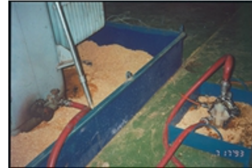
Photo : Temporary bunding for transformer decanting
