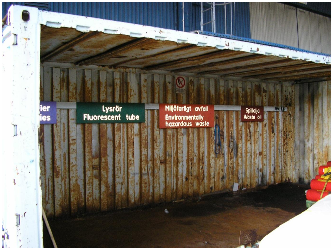
Simple covered storage area for hazardous materials using an ISO container with one side cut away.
