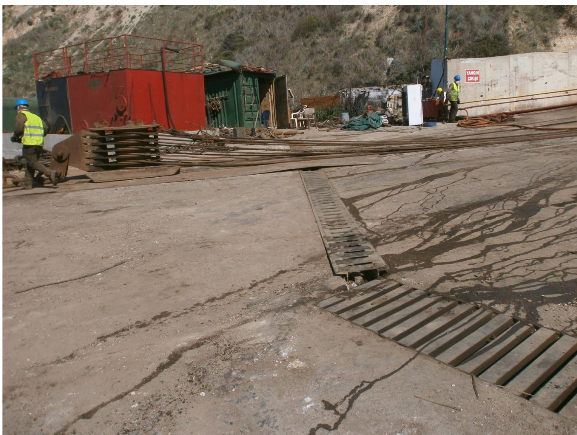
Hard standing with drainage channels.
