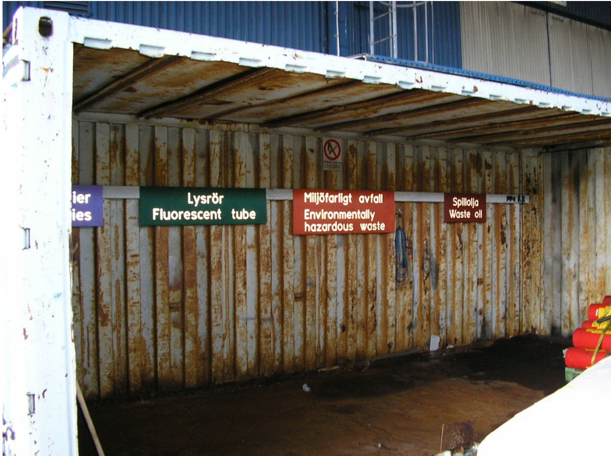
Figure 2- Simple covered storage area for hazardous materials using an ISO container with one side cut away. Photo: R Watkinson
