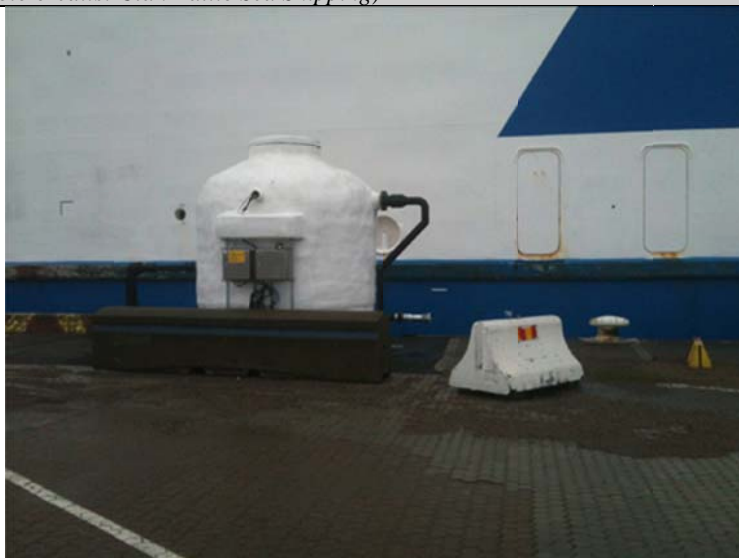
Example of a facility for the direct reception of sewage in the port of Trelleborg (Sweden) (Photo credits: Clan Baltic Sea Shipping)
