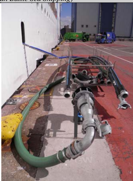
Example of a facility for direct collection of sewage in the port of Helsinki (Finland) (Photo credits: Clean Baltic Sea Shipping)
