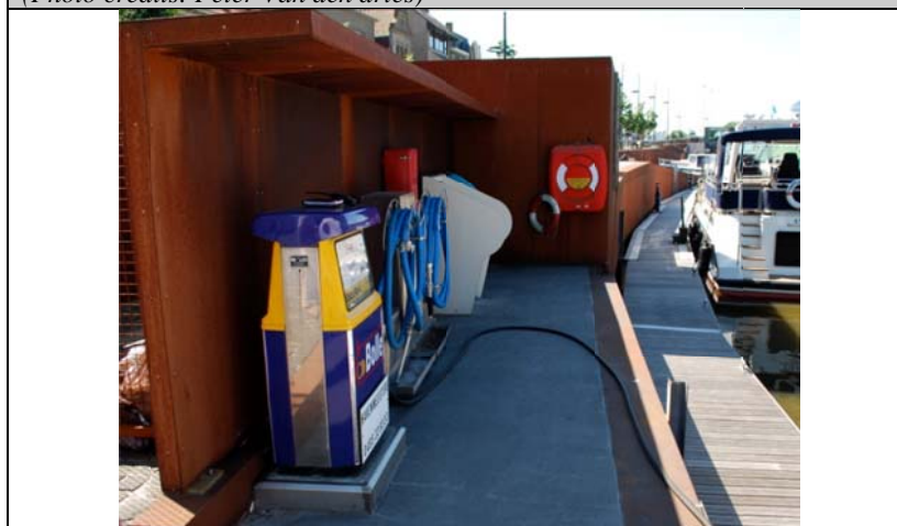
Example of a combined reception facility for bilge water and garbage in a recreational port (Photo credits: Peter Van den dries)
